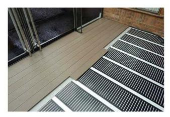
We can set this temperature higher or lower simply by raising or lowering the voltage at which the system runs.
